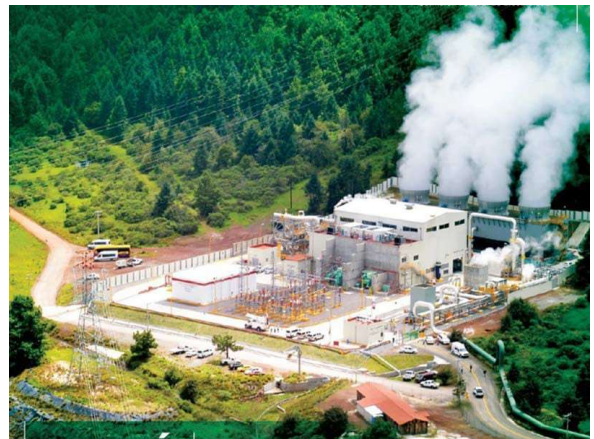
Pathé Geothermoelectric Power Plant, Hidalgo | CFE.
