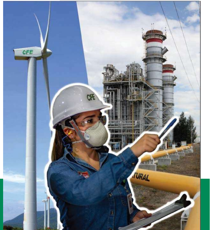
Wind power plant, La Venta, Oaxaca, CFE.
