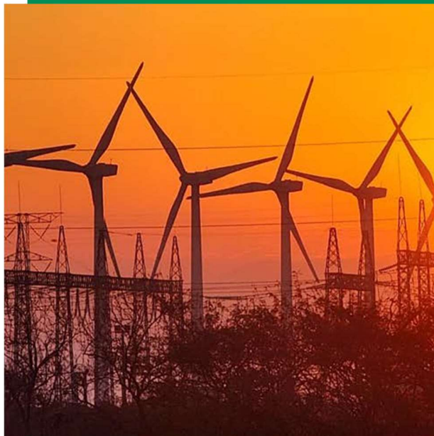
“La Venta I y II” Wind Power Plant, Oaxaca | CFE.
