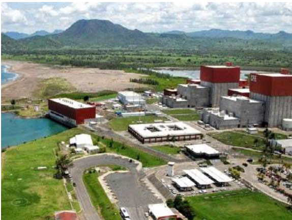
Laguna Verde Nuclear Power Plant - Veracruz | CFE.
