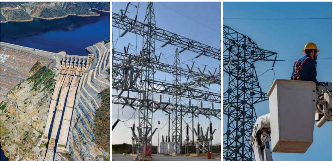
La Yesca hydroelectric power plant, Nayarit | Saltillo electrical substation, Coahuila | Electrical tower maneuvers, Sonora.
