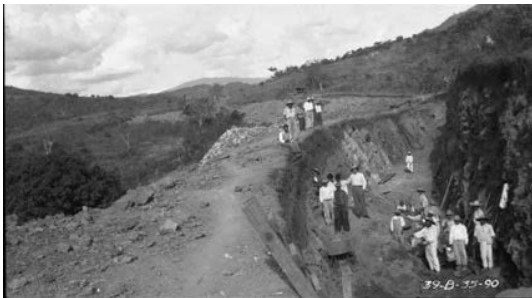
Infrastructure of Ixtapatongo, first hydroelectric power plant | CFE.
