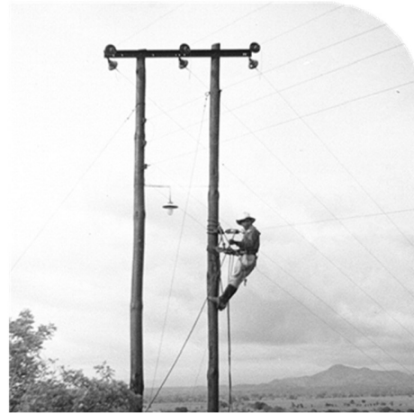
Image: Liniero maneuvering on energized line | CFE
