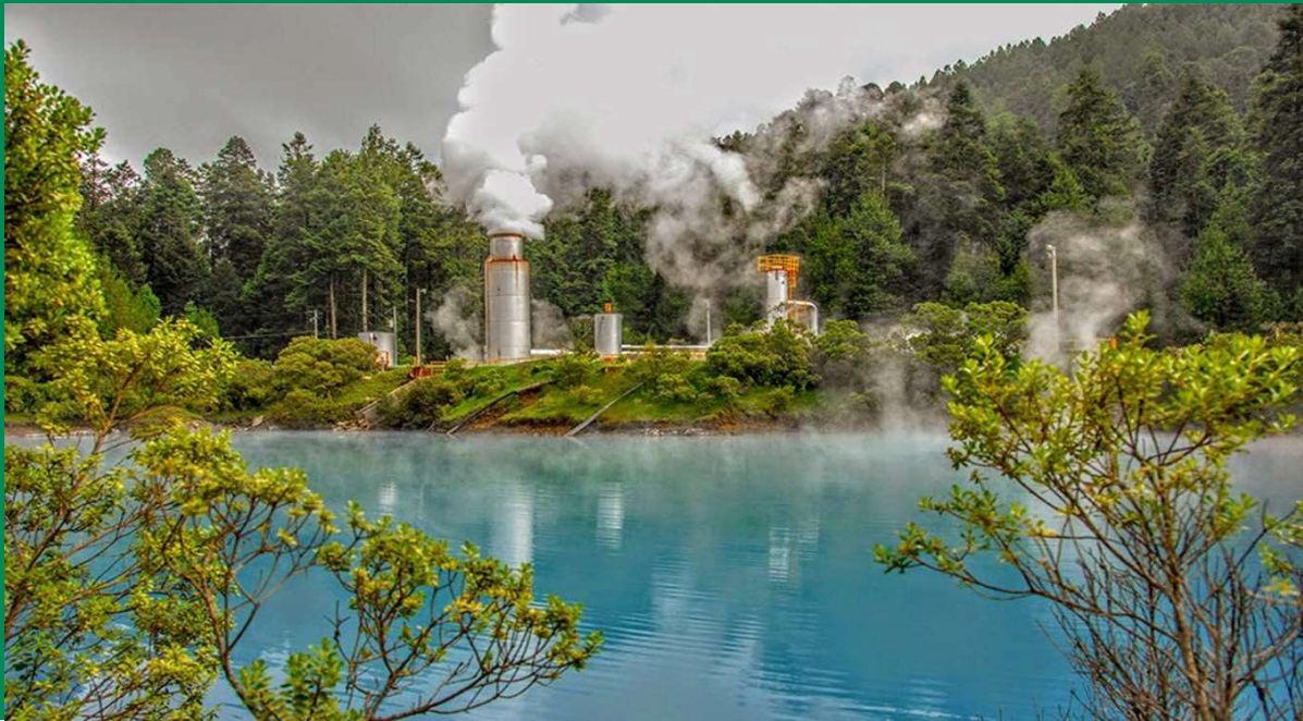
Image: Los Azufres geothermal power plant, Michoacán, CFE. Certified by the PROFEPA with the distinctive Clean Industry.
