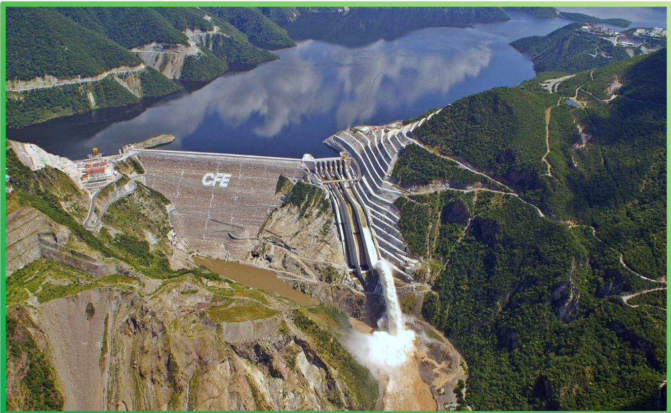
CFE's Hydroelectric Plant Ing. Alfredo Elías Ayub (La Yesca)
